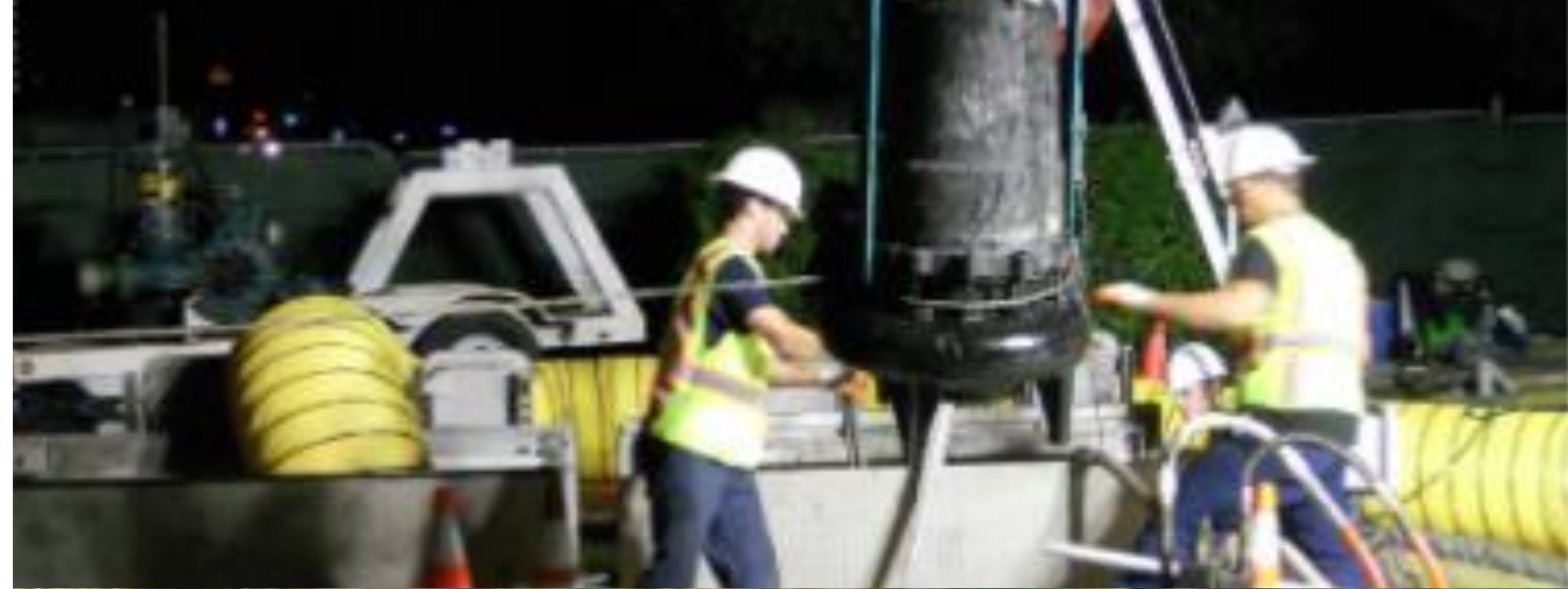
Glorietta Bay Pump Station Improvements – City of Coronado
