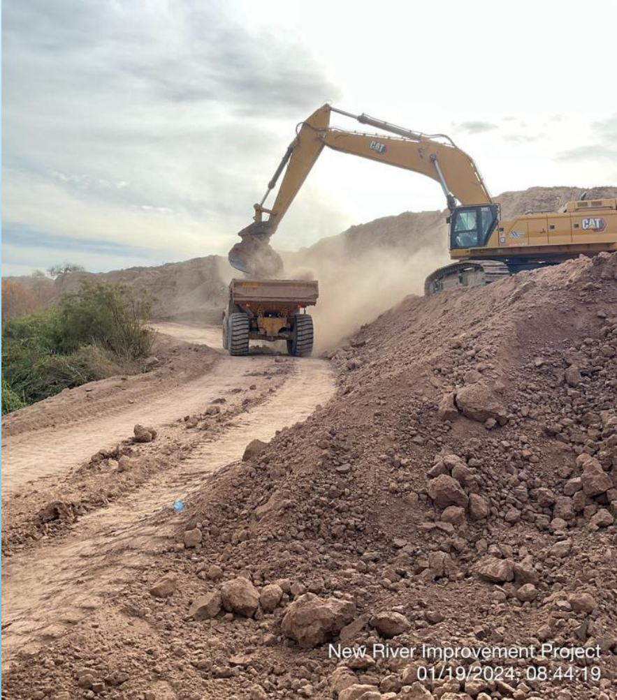
01/19/2024 Excavating along slope area & rock trucks hauling to lay down yard
