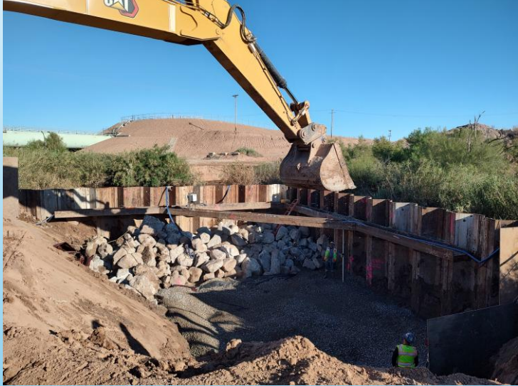
Rock & structure pad within cofferdam, 3/2024
