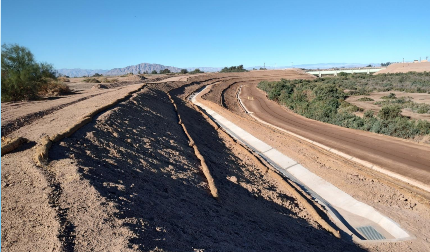
11/18/2024 top slope looking west
