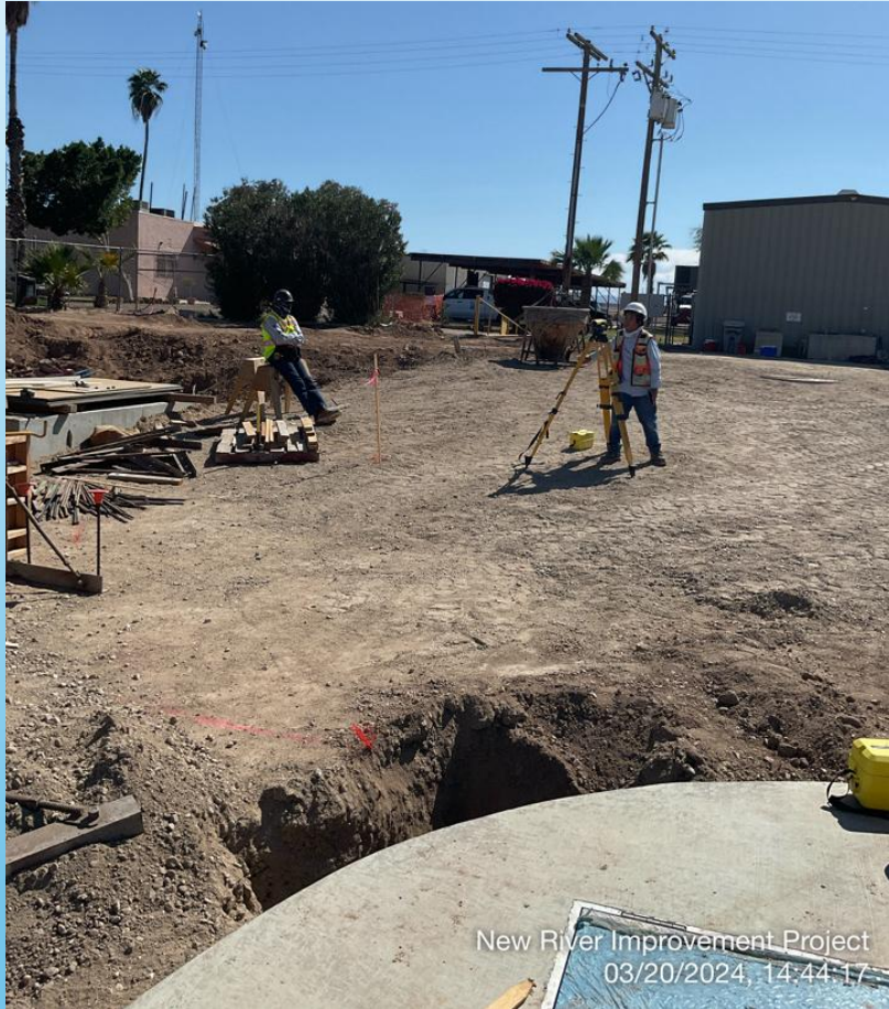
03/20/2024 forming pump pads, checking grades
