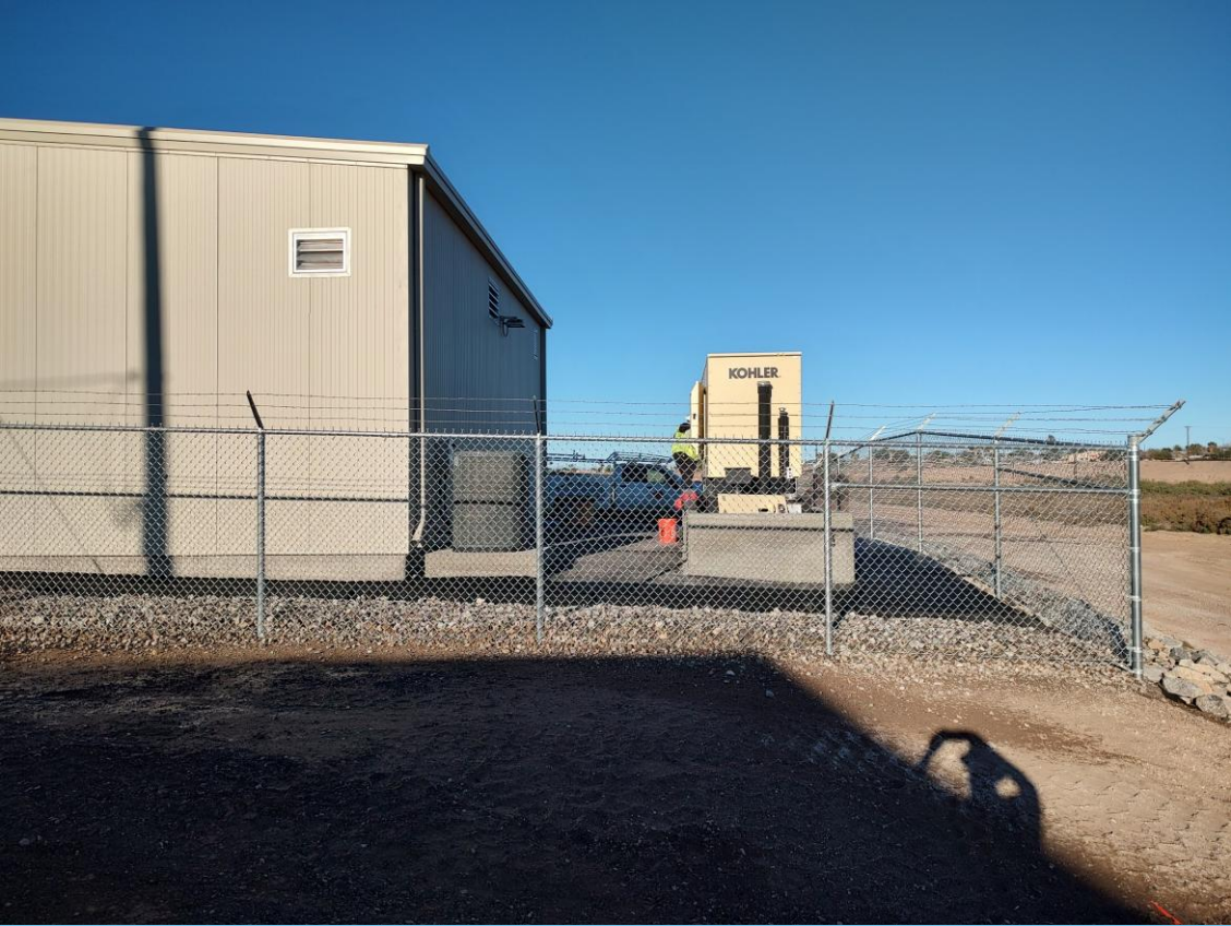
01/13/2025 8' CL fencing & rock backing in place
