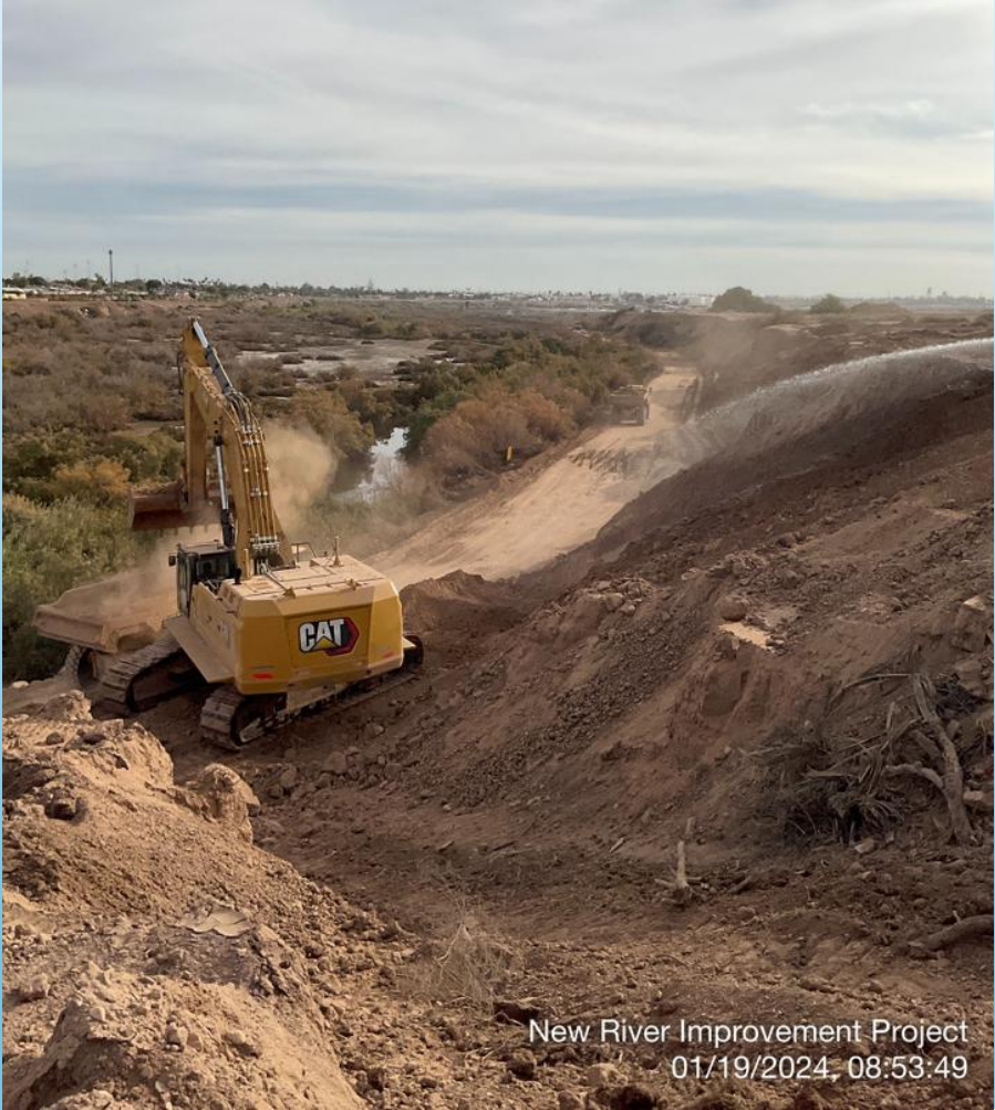
01/19/2024 Excavating along slope area & rock trucks hauling to lay down yard
