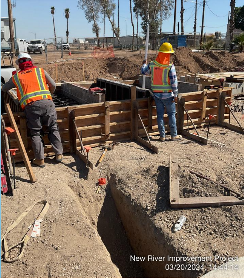
03/20/2024 forming pump pads, checking grades
