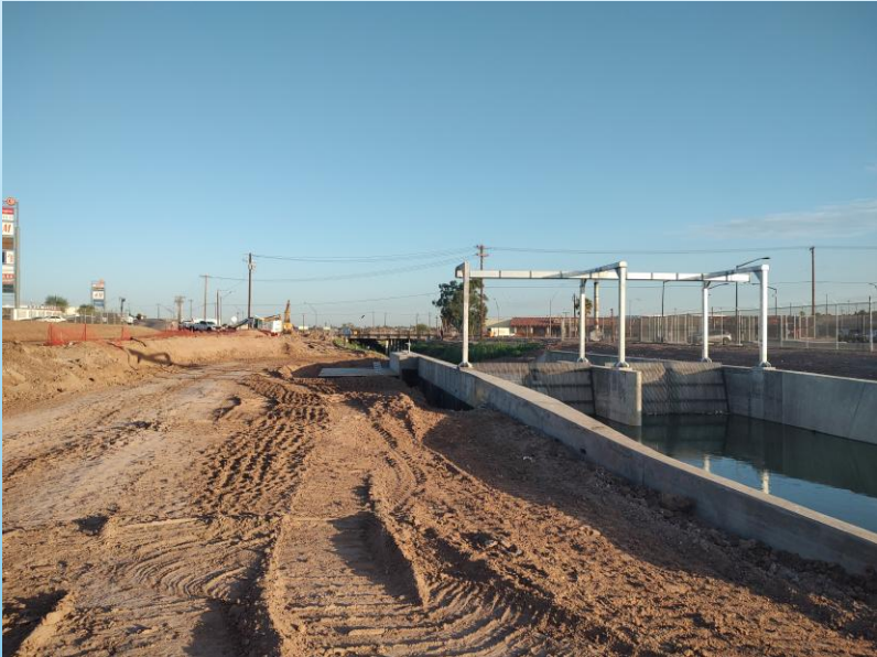
Looking NW, Temporary Diversion Removed, Area Filled and Compacted
