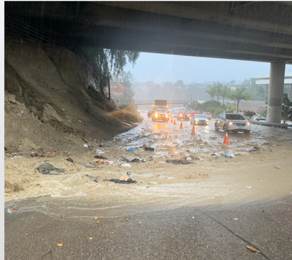
Erosion and mud slide during 2020 rain event due to stormwater pipe failure near 163
