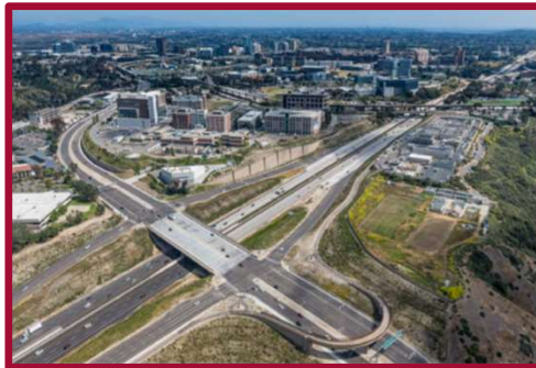
Highway City of San Diego, I-5/Genesee Avenue Interchange
