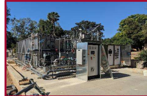
Utilities SD Zoo Safari Park, Wastewater Treatment Plant Expansion
